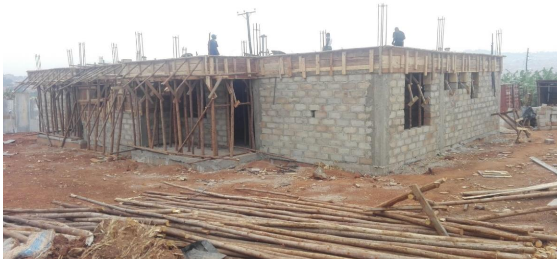
Figure 6 : Construction of staff housing
