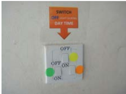
Color coded power switch for power saving
