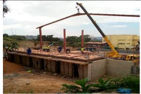
Figure 15Laying the steel reinforcement bars and hollow clay blocks for the first floor slab and fixing the steel portal rafters
