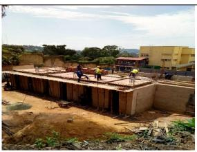
Figure 12 Fixing the formwork for the first floor slab
