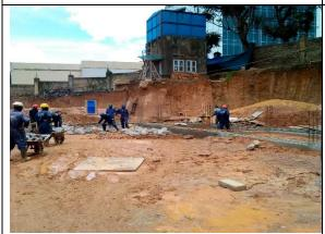
Figure 7 Casting the reinforced concrete ground beam and soil backfilling in foundation
