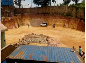
Figure 2Excavation of the soil to reduce levels
