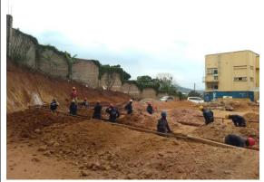
Figure 3Excavation of the foundation trenches of the store
