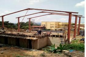
Figure 16 Casting the reinforced concrete slab for the first floorand fixing the steel portal rafters
