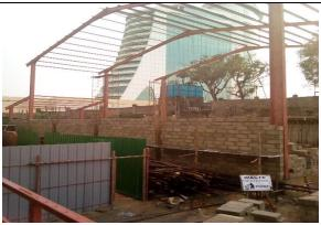
Figure 18 Fixing the mild steel Z-section purlins
