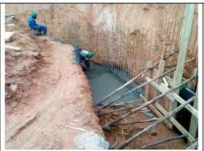
Figure 5Casting the reinforced concrete retaining wall base
