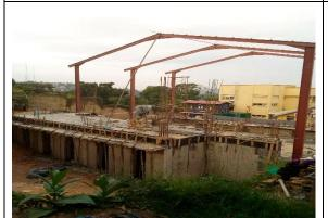
Figure 17 Reinforced concrete slab for the first floor
