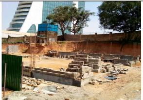
Figure 10 Construction of concrete block walling for the ground floor
