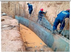
Figure 6Casting the reinforced concrete retaining wall
