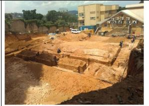
Figure 4Excavation of the foundation trenches of the store
