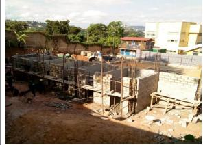
Figure 11 Construction of the concrete block walling for the ground floor
