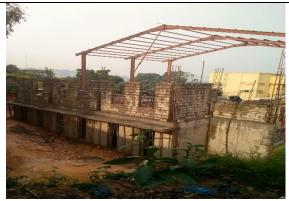
Figure 19 Construction of the concrete block walling for the first floor
