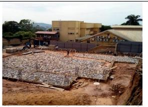
Figure 8Hardcore filling in the foundation
