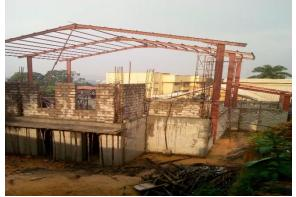
Figure 20Fixing the mild steel Z-section purlins
