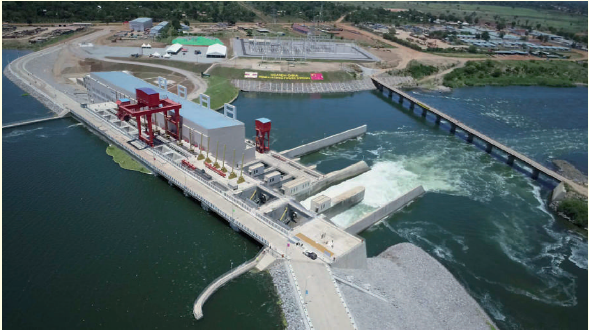
Isimba Hydropower Project located on the border of Kayunga and Kamuli districts
