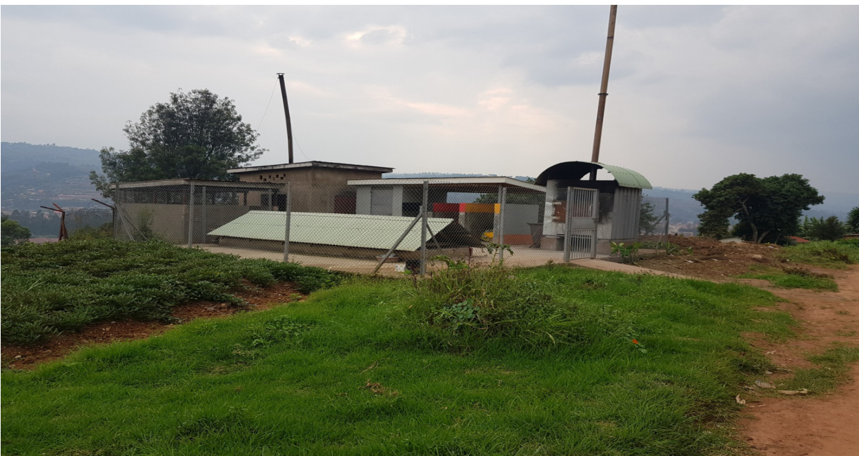
Figure 8.6: Waste disposal area enclosed in a chain link fence with gate (Source: Kagga & Partners)
