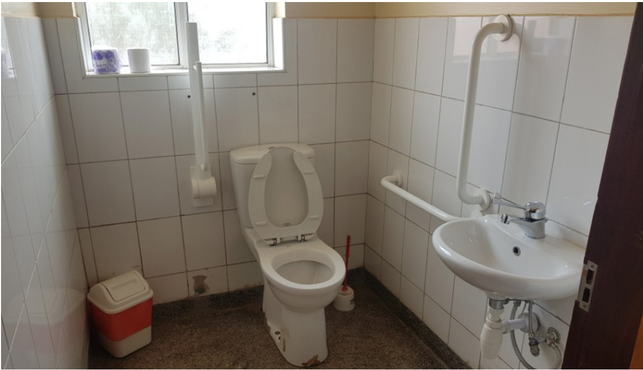
Figure 4.7: Water borne toilet (seat type) with grab rails for persons with disabilities with a hand washing facility within reach of the user
