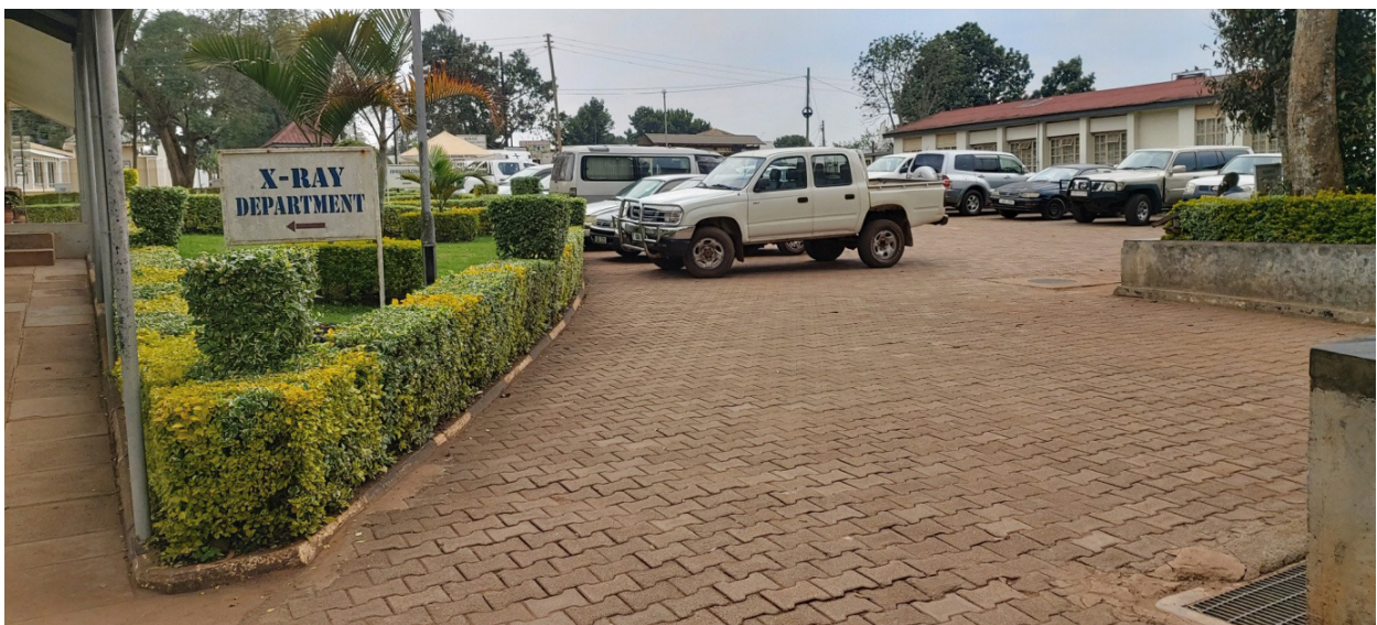
Figure 10.3: Good landscaping; Paved parking space with clear signage
